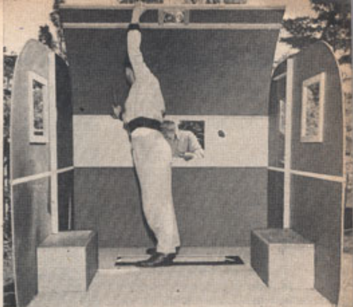
Top curves into place after side walls and front bulkhead have been attached. All seams are caulked to keep out water. Sides and top are composition board, reinforced with wood.
